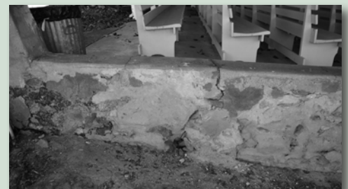
Water damage is eroding floors and foundations.
